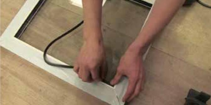
**7** Take the wedge gasket and starting at the corner push it in between the glazing and aluminium vent.
