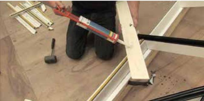
**3** Silicone the foam board securely into place.
